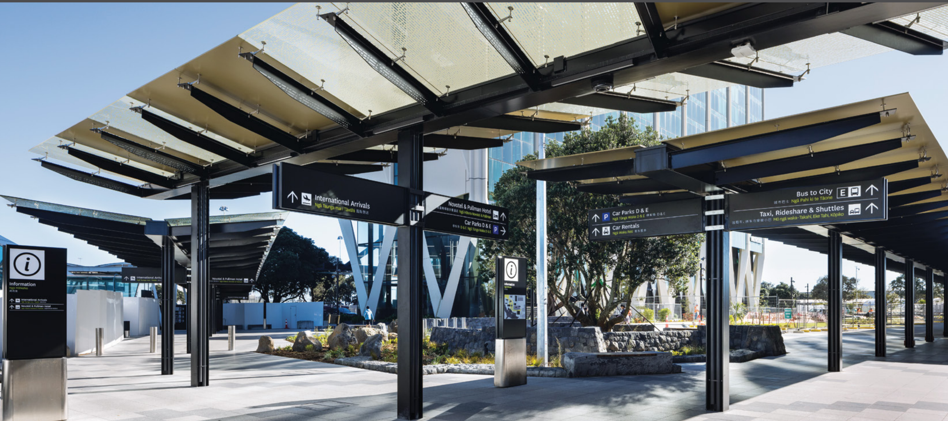
Auckland International Airport Walkway | Auckland, New Zealand
