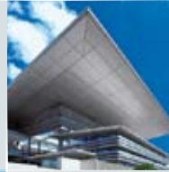
Australia Auburn Power Centre, Shopping Centre
